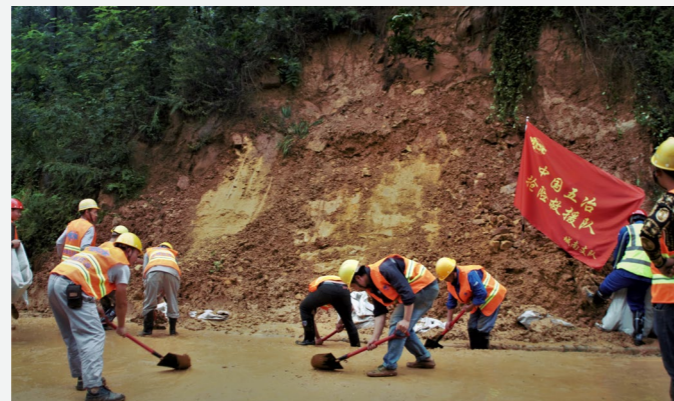
Disposal of landslides and road maintenance by MCC5
