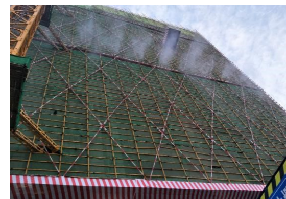
High-altitude spray dust reducing
