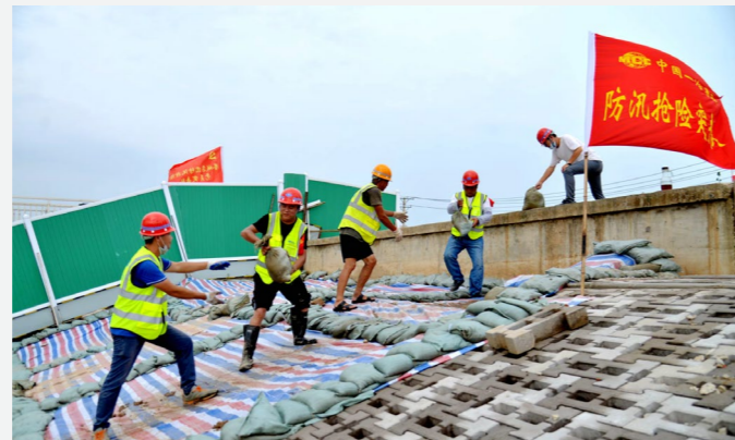
CFMCC reinforced slope protection at Hongshan river beach in Wuhan
